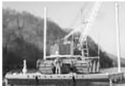
32' x 40' x 4' Sectional Spud Barge and Crane.
